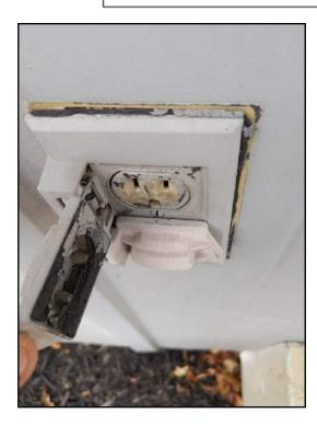
DISTRIBUTION SYSTEM \ Cover plates Condition: • Missing
